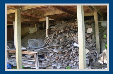
No deck, regardless of the material used to build it, would be safe if this amount of fuel beneath the deck caught fire. Even decks that may have a noncombustible surface, such as light-weight concrete, use lumber and timbers for structural support and those materials can catch fire.
