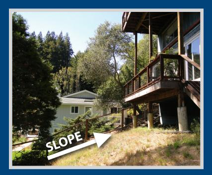
Managing vegetation on the slope is important for reducing the exposure to the deck and minimizing the chance of ignition from a wildfire. Fire burning up the slope to the deck can expose the bottom and side of the deck to heat, flames and embers.
